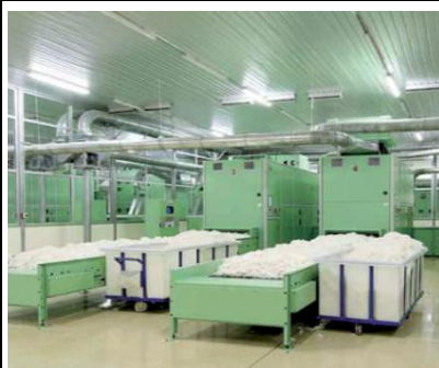
Machinery Name: Blow room
